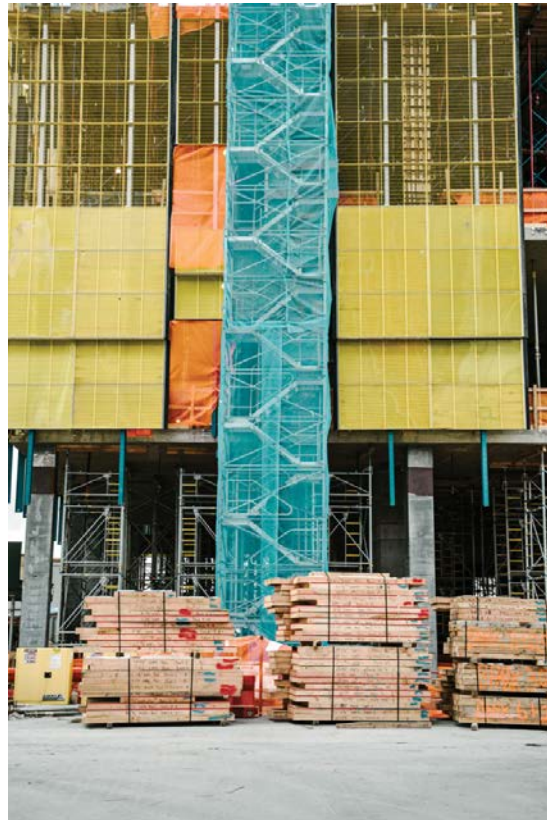
The temporary stair tower at the base of 35 Hudson Yards, the site's only mixed-use tower. Photo courtesy of Joshua Scott
